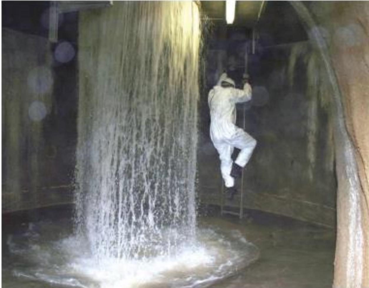
Fig. 8. Circular water jet falling down into the energy dissipation chamber of the Wiggan drop shaft during a minor rain event. The total drop head is 11.2 metres. (Photo: Hohl)
